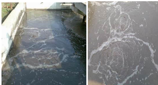
Figure 2: PTIGN upgraded aeration basin
